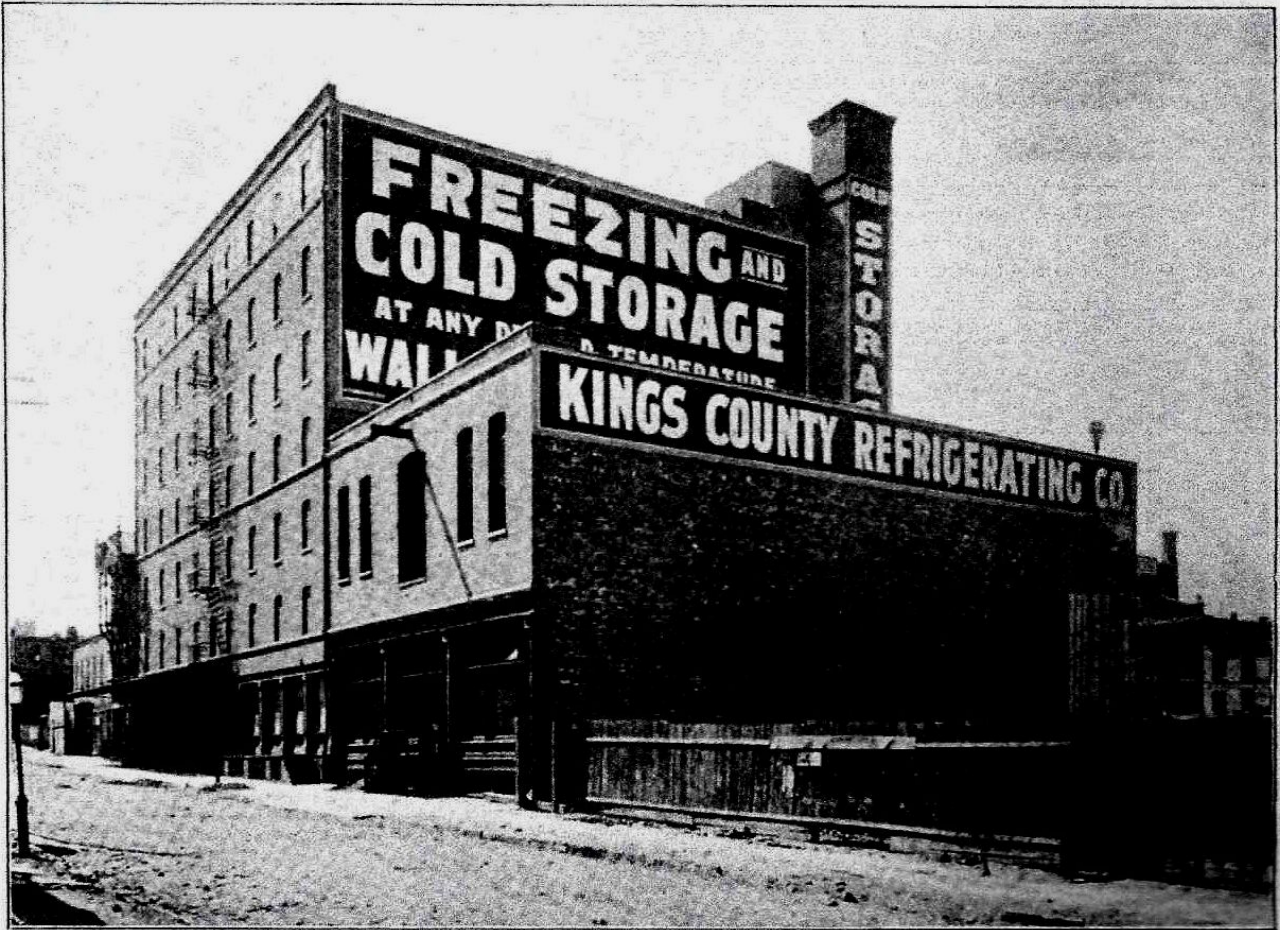
WAREHOUSE AND POWER HOUSE. KINGS COUNTY REFRIGERATING CO., BROOKLYN, N. Y.
